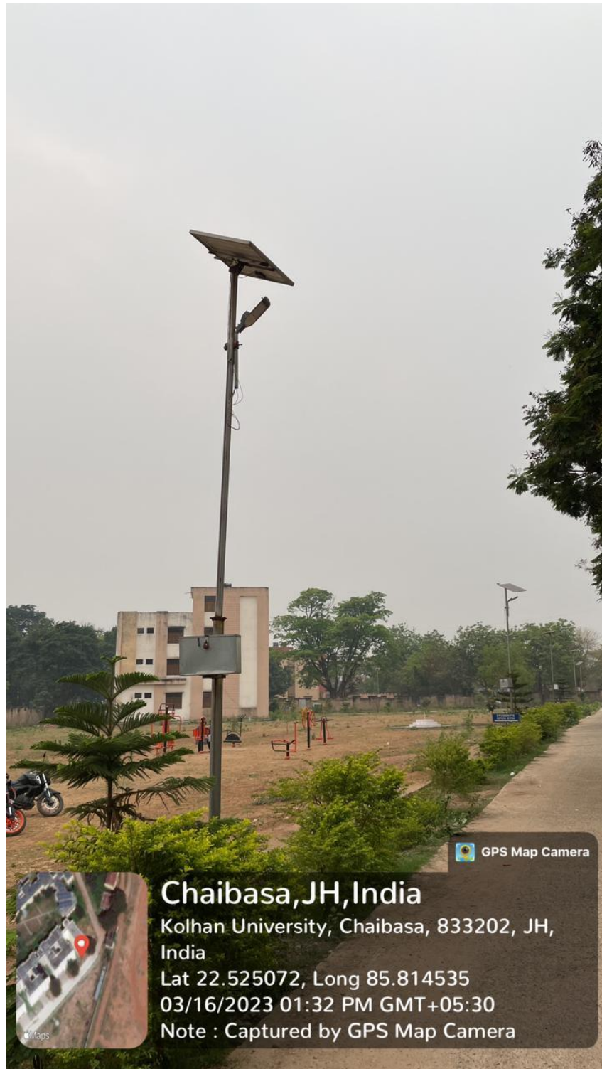
Figure: Solar energy powered LED street lights in the university campus
